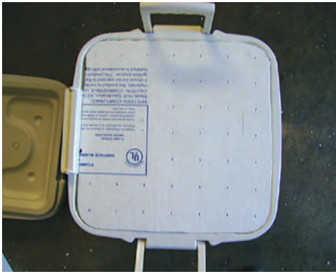
Check the fit and cut more if necessary. This piece will be slightly rectangular, so mark it directionally, I mark it where the notch (back) side is.
