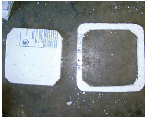
Cut a square out of the middle, about 1"-1.25" from the edge. Save the cutout for later. Notice the directional markings on the left.
