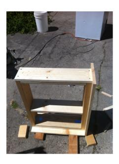
on the collar. The 1x10 length will be the same length as the sides of the collar. I glued and nailed them the same as the first board and finally put the last board on the back section.
