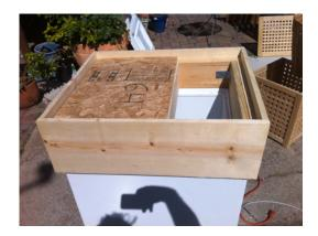
Measuring the inside area to the center of the 1x6 middle support, I cut a piece of plywood to fit. In my case, I again some ugly particle board on hand, so I simply purchased a small piece of nice quality ¼ inch finished plywood to go on top of my ugly particle board. I could have just bought half inch quality plywood, but again, I was spending less on material and more on time.
