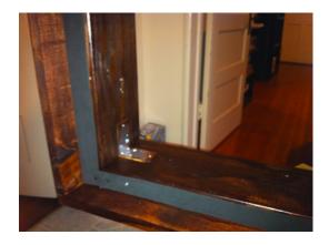
I gave everything a nice stain and several coats of polyurethane. After it was all dry I tacked a bit of neoprene around the bottom edge to give it a real good seal and eliminate the minor wobble from running the temp probe over the edge of the freezer.
