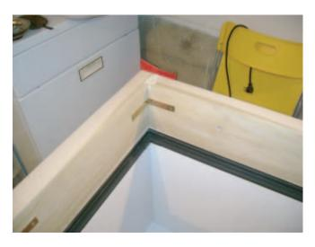
We reinforced the inner corners with brass brackets, and you can see the wood filler that i used to make the seating surfaces perfectly smooth.
